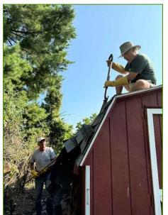
You might have noticed Alan Farr, Jim Richardson and Rob Todd on the shed roof at the Village Hall recently. Well, they aren't just "fiddling on the roof." They've taken on the task of replacing the weathered shingles on the shed roof.
